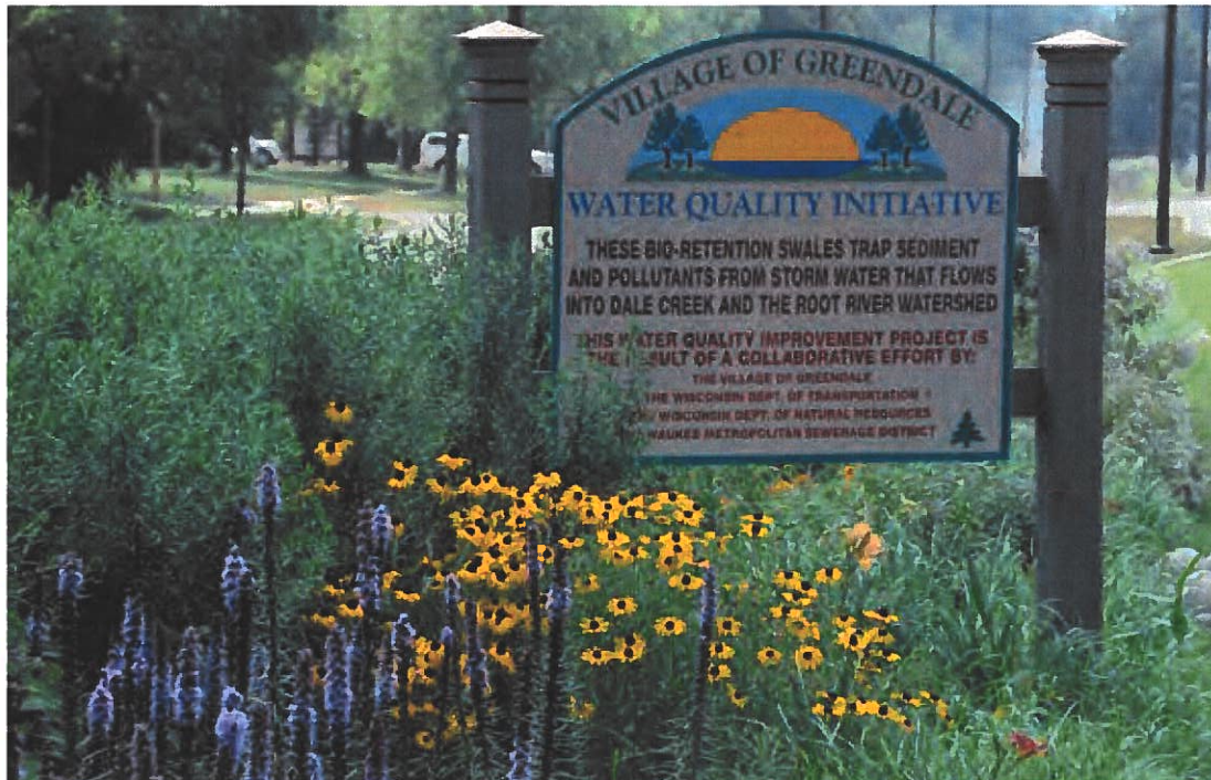
The Grange Avenue green street uses bioswales to capture roadway stormwater runoff. It slows down the stormwater runoff rate and removes pollution, while providing an attractive natural setting to the busy roadway
