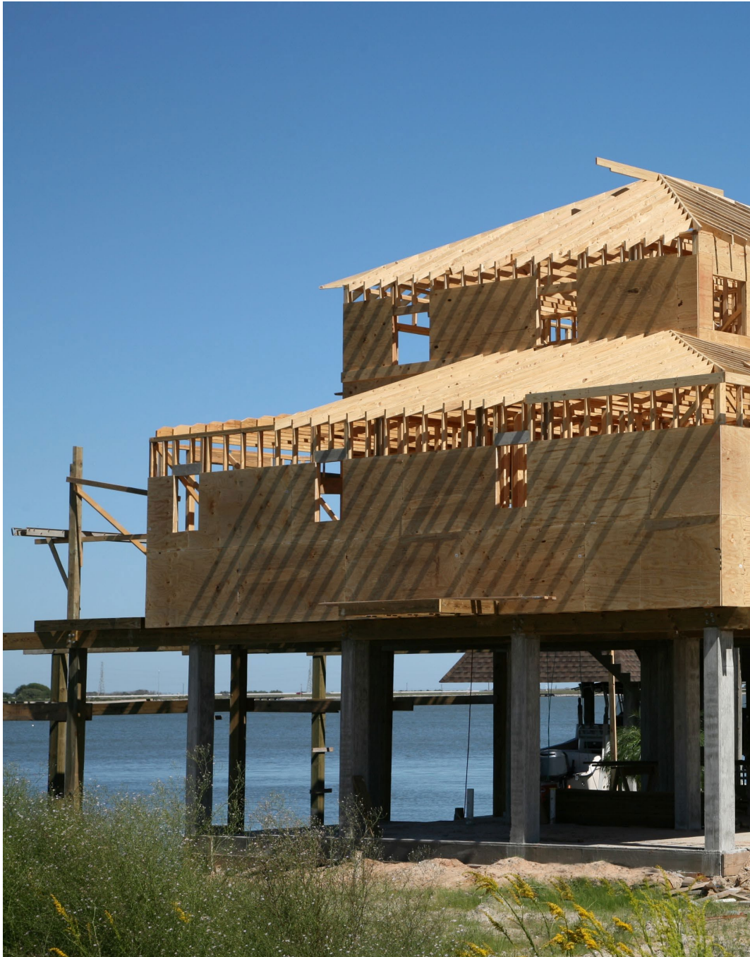
An elevated coastal house in the process of being built
