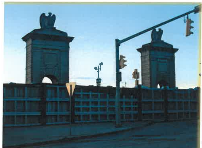
Figure 10: Flood Walls along Market Street, Wilkes-Barre, Pennsylvania
