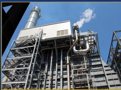
Duke Energy's gas-powered plant, Masontown, Pennsylvania.
