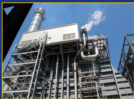
Duke Energy's gas-powered plant, Masontown, Pennsylvania.
