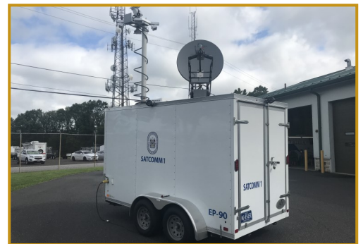
Satellite communications trailer ready to deploy anywhere in the region.
